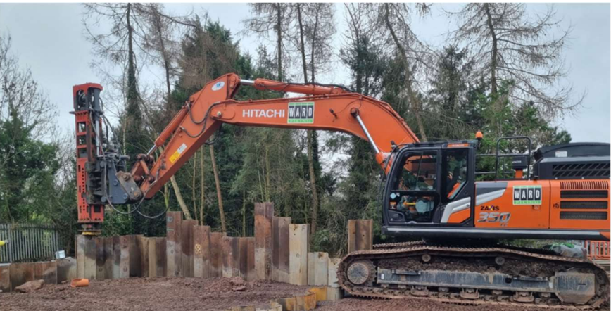
Hitachi and Movax DH25 impact hammer at working radius of 7.5m from front of tracks
