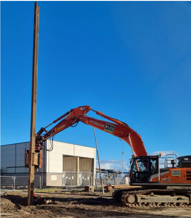
Hitachi and Movax SG75V at working radius of 6.5m from front of tracks
